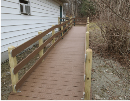
New handicapped access ramp
