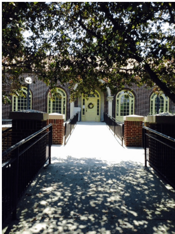
The completed ramp into the Library
