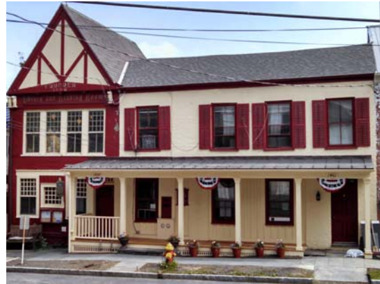
A covered access ramp was installed
