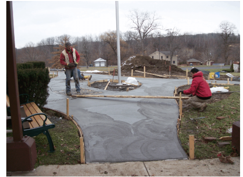
Building an outdoor space
