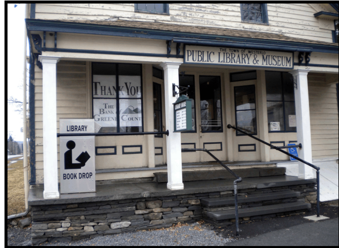
The new book drop on the left side of the porch
