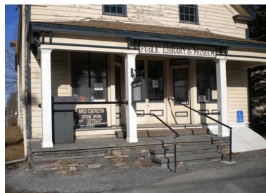
Porch completed with new wood columns
