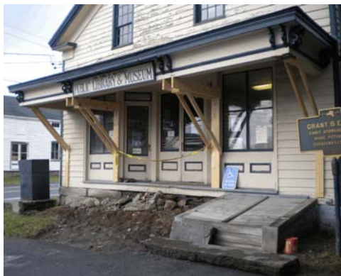
Porch under construction
